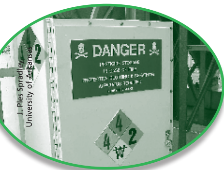
A National Fire Protection Association (NFPA) warning on a storage box for fumigants. The strikeover on the letter W in the white diamond alerts firefighters not to use water to put out a fire.
